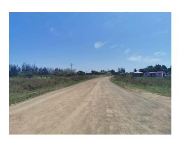
The objective of the project is to re-gravel of P425 from km 13 to 20 km. There is no gravel left on the current surface and is slippery when it rains the road requires new gravel surface layer to be placed.
